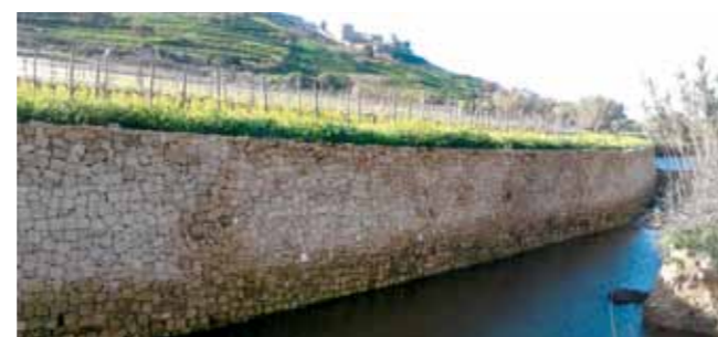
Construction of the rubble walls at Ramla Valley in Gozo in the framework of the Alter Aqua Programme, September 2013.
