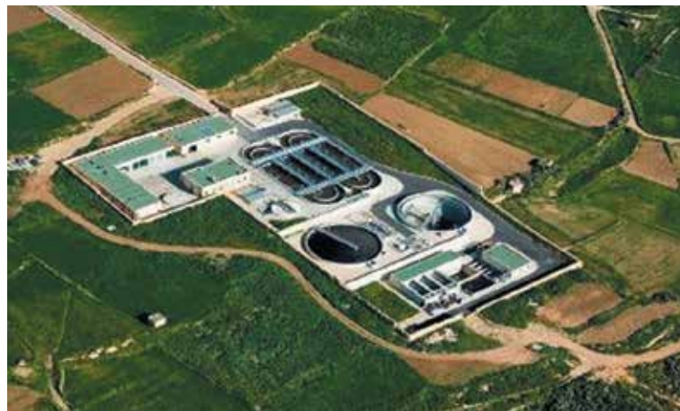
Aerial view of wastewater treatment plant at Ras il-Hobż, Gozo © Department of Information, Malta
