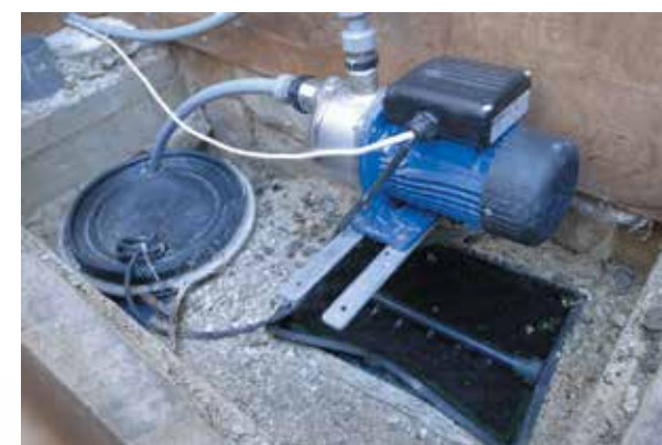
Close view of greywater treatment system personally assembled by Eng Marco Cremona for his house in Malta © Rene Rossignau
