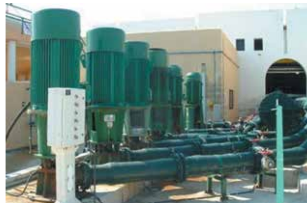
Reverse Osmosis installations
